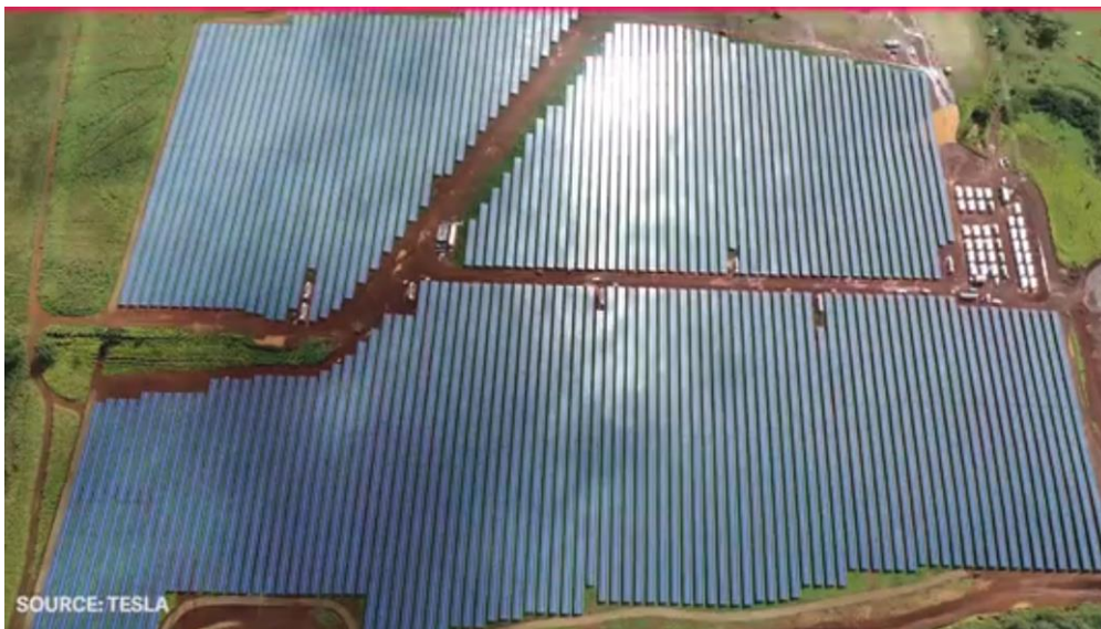
13 megawatt solar farm and 52 megawatt-hour battery storage on 50 acres
