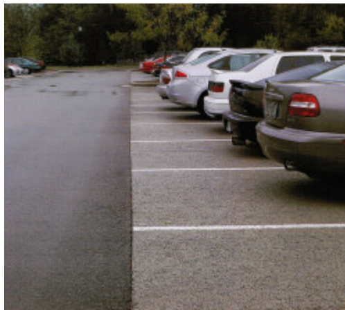
Paving with Pervious Concrete by George Garber, P.25.
