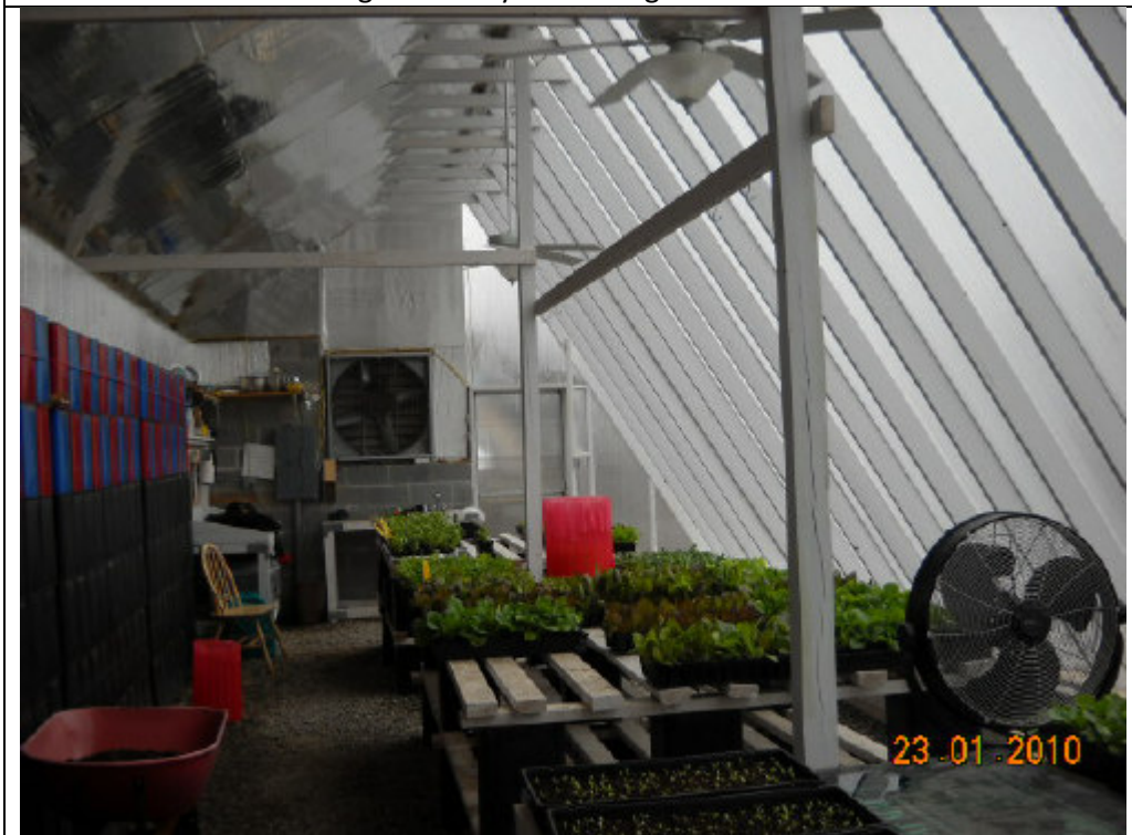
Note the use of rectangular honey cans along the north wall for the heat sink.
