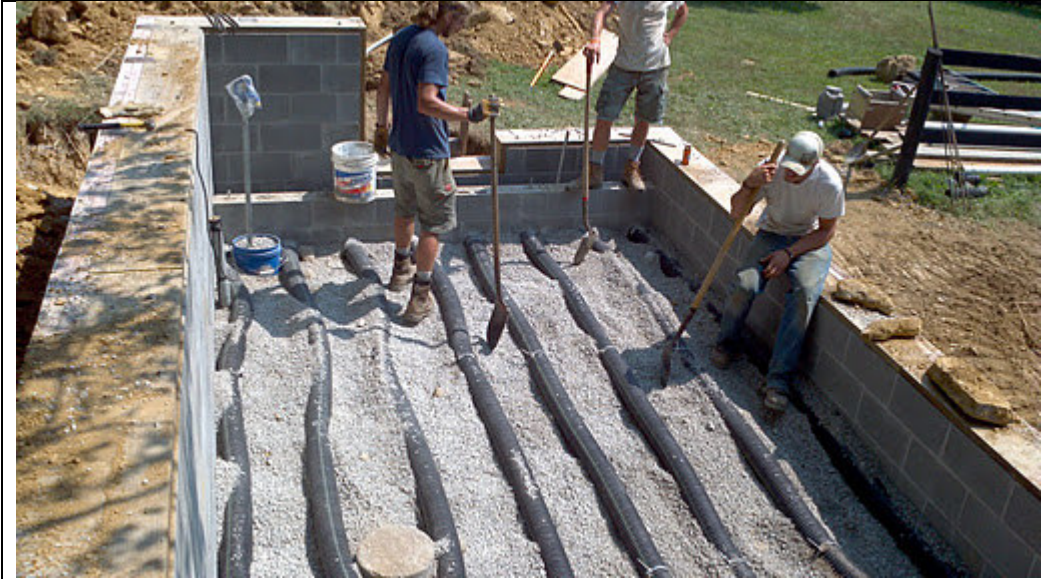
The last layer of pipes is covered with rocks.
