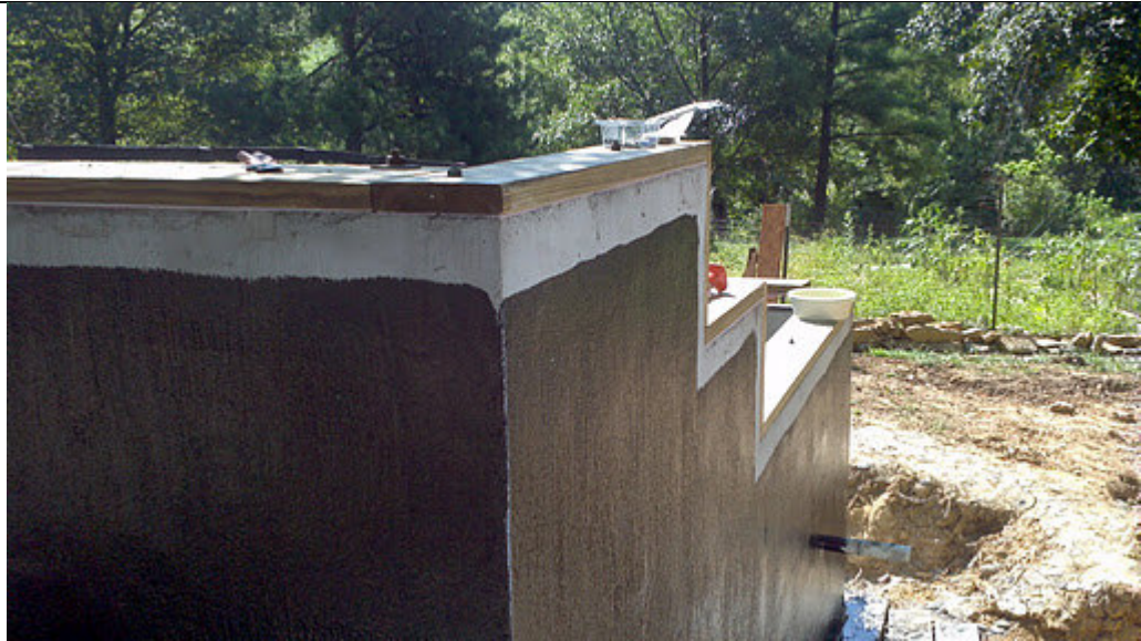
Waterproofed outside walls.
