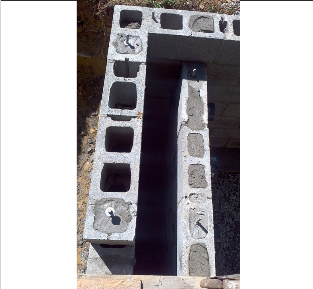
This shows the plenum that draws air into the 24 heat-sink pipes.
