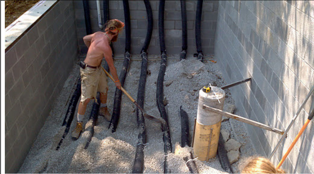
Starting to install the 24 heat-sink pipes.
