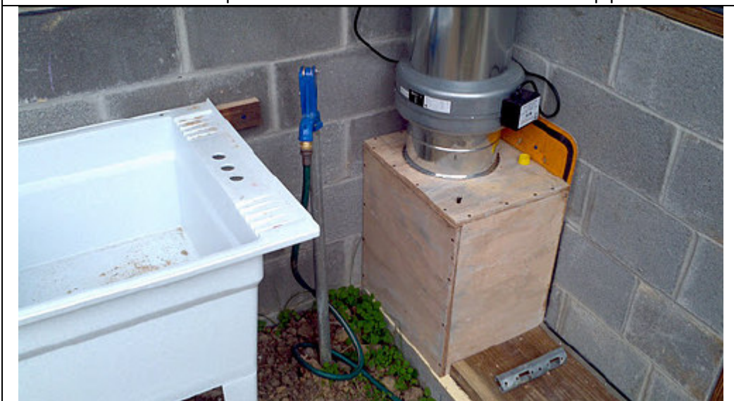
Cover of the plenum of the heat sink and fan to push air into the plenum.
